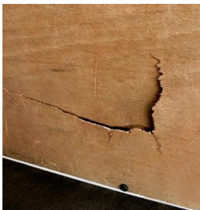
Painel lateral rachado
